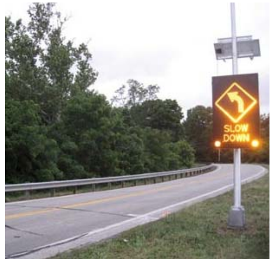
Image 3: One type of dynamic curve warning system
