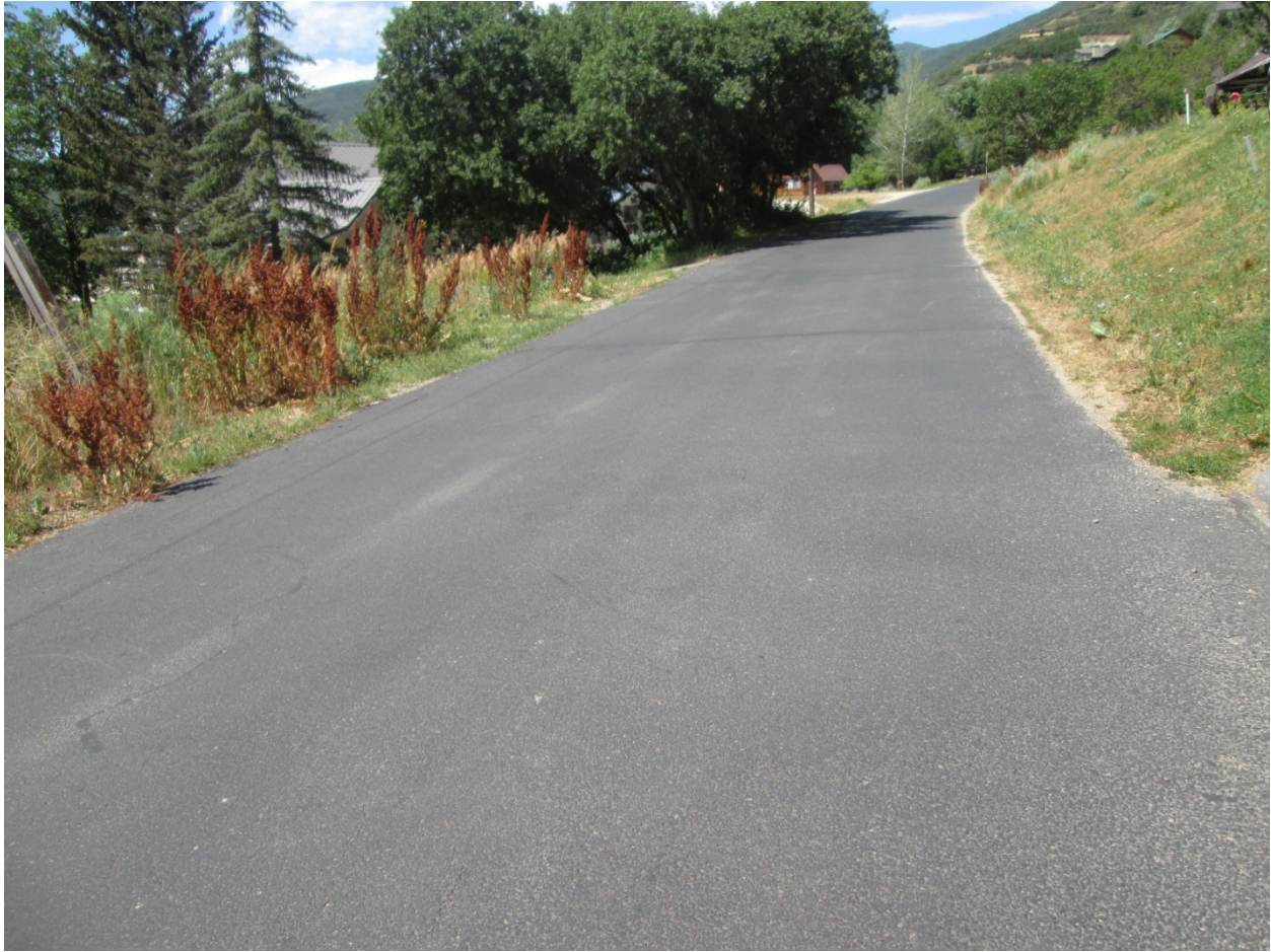
Photo 2. Good Condition – Interlaken Dr from Interlaken Dr to Luzern Rd (RSL = 10 years)
