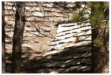
This home has a triple threat: wood shake roof, pine trees overhanging the house, and dead needles and other debris collected on the roof.
